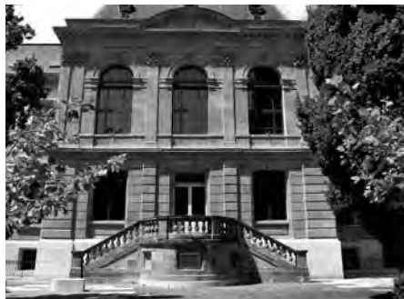
Figure 1: The main University building was energy retrofitted with special attention to its high architectural value.
